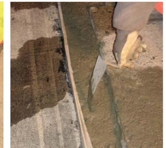
Maintenance works in Malpensa: requalification of tested slabs and joints of the 17L/35R runway
