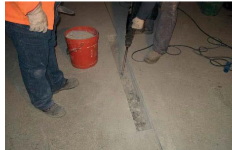
Maintenance works in Malpensa: requalification of tested slabs and joints of the 17L/35R runway
